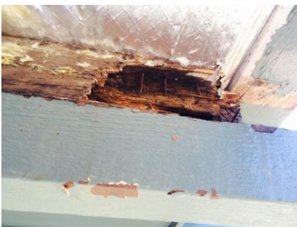
Floor joists that needed reinforcing
